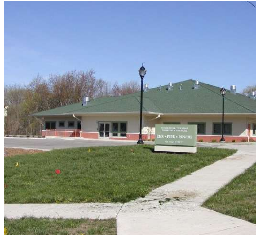
Emergency Services Building built in 2004
